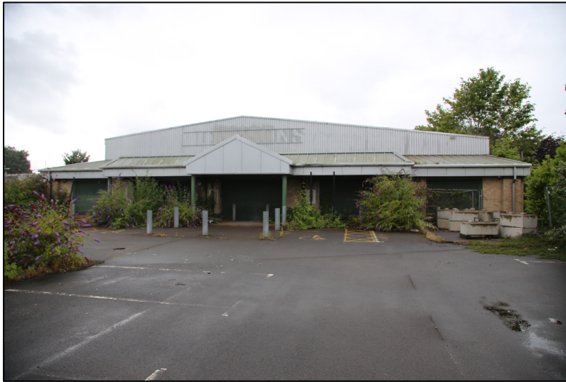
Existing building condition
